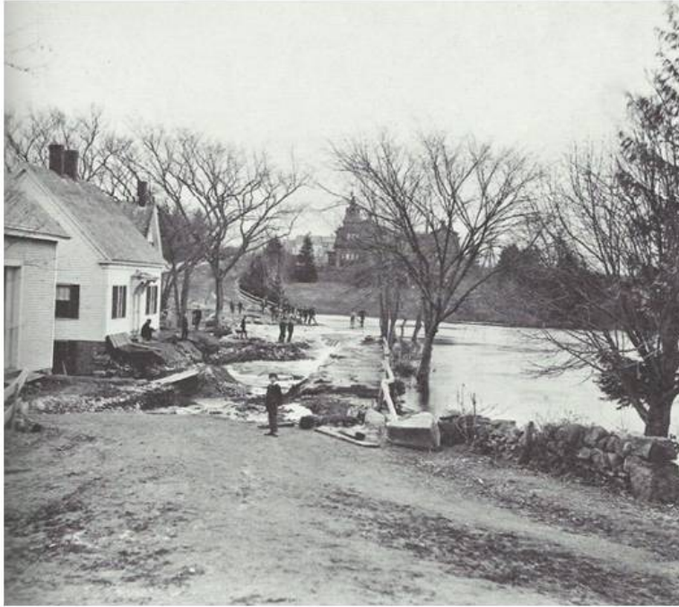
Figure 12: Flood of 1891. Source: John A. Dennehy, P39.
