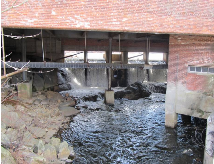
Figure 25: Hollingsworth Dam at Armstrong Factory. Photo by Benjamin D'Agostino.
