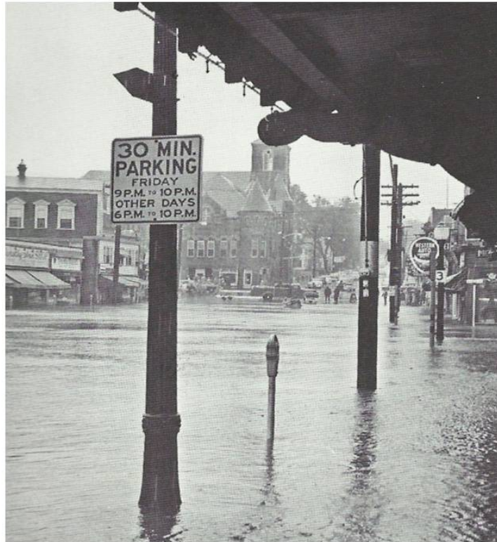
Figure 14: Flood of 1948. Source: John A. Dennehy,P36.
