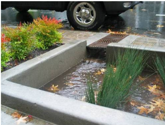
Figure 30: Sidewalk before (upper left) and after implementation of BMPs in Portland, Oregon. The BMPs incorporate curb cuts and filter strips to collect street runoff and allow infiltration into the soil. Educational components are implemented through interpretative signage so that the public will be aware of the project goals and objectives of reducing the flood risks and the amount of runoff entering catch basins. Source: ASLA 2006 Professional Awards.
