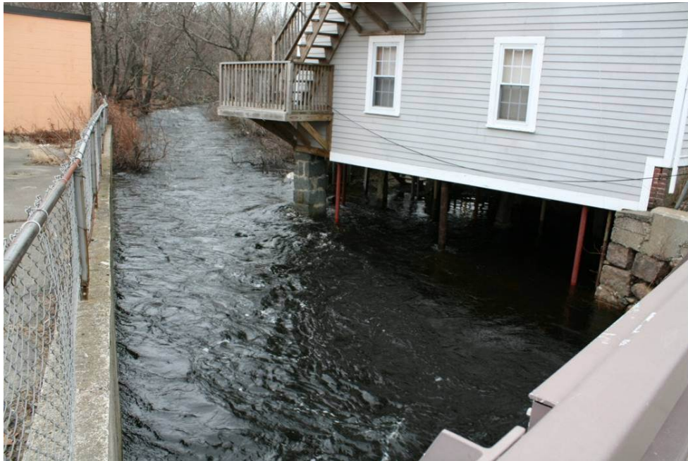
Figure 82: House on stilts at the Adams street bridge showing the Monatiquot River running 4 feet under the home. Photo by Elizabeth Englebretson, 2011.
