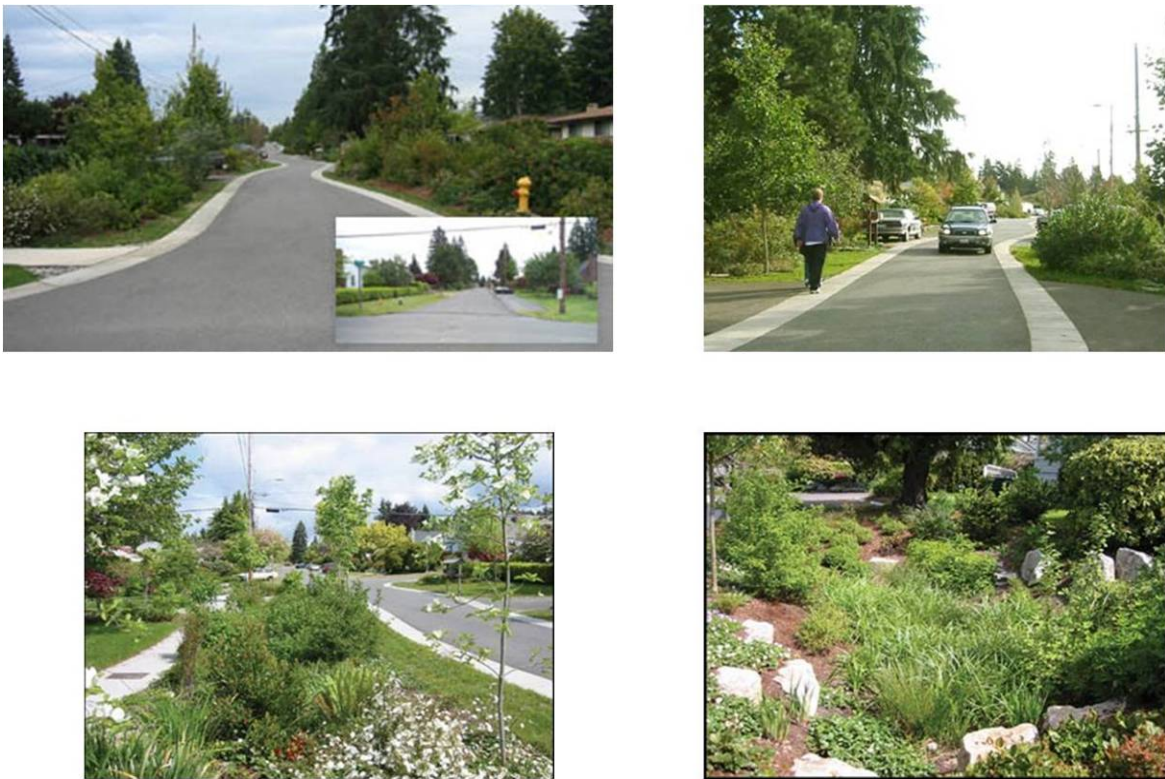
Figure 31: SEAStrEet demonstration project of stormwater management practices along the street in Seattle, Washington. Meandering streets provide safer streets that encourage mobility. Stormwater management techniques along the street promote infiltration such as bio-retention swales. Source: City of Seattle.
