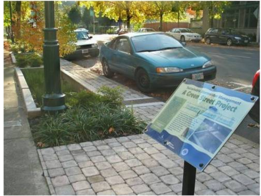
Figure 30: Sidewalk before (upper left) and after implementation of BMPs in Portland, Oregon. The BMPs incorporate curb cuts and filter strips to collect street runoff and allow infiltration into the soil. Educational components are implemented through interpretative signage so that the public will be aware of the project goals and objectives of reducing the flood risks and the amount of runoff entering catch basins. Source: ASLA 2006 Professional Awards.
