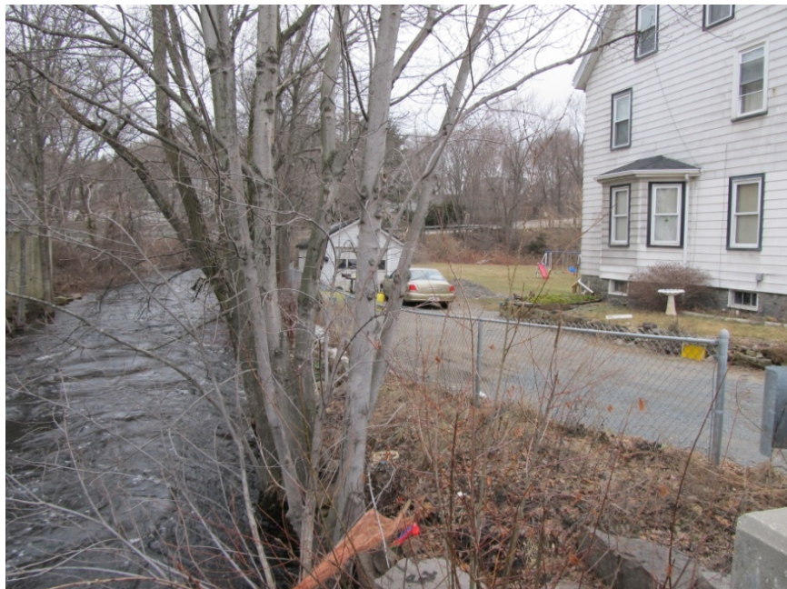
Figure 37: Close proximity between residential property and Monaquot River on Adams Street. Photo by Benjamin D'Agostino.
